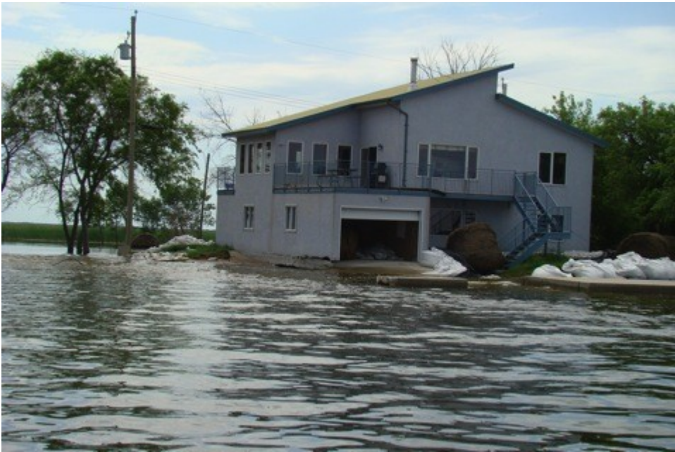
Destruction after May 31 st storm:
